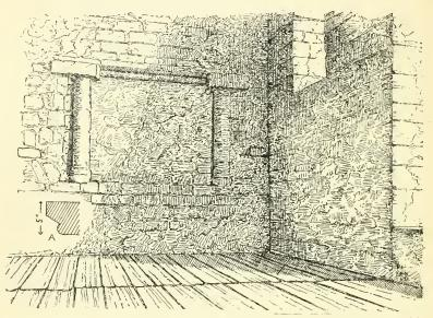
F1G. 93.—Recess in chamber in the western tower at Skipwith, Yorkshire. At A is the section of the lintel of the recess.
