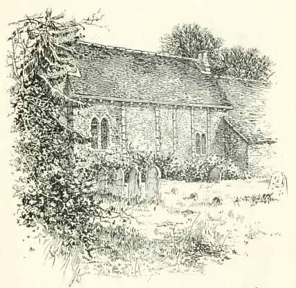
F1G. 36.—Pilaster strips on the nave wall of Woolbeding Church, Sussex. The strips are about 7 in. in width.
